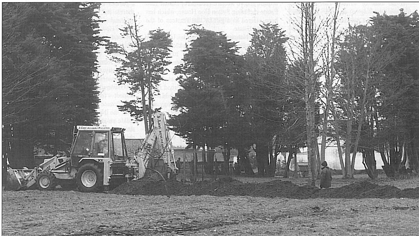
Archaeological trial trenching at Sutton Hoo House in February 1997. The work was undertaken in advance of the construction of the proposed Visitor Centre by the National Trust (Photograph: Suffolk County Council)
