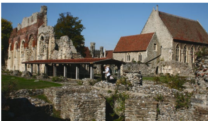
The modern roof (centre) over the Porticus of St Gregory, the original burial place of the first seven archbishops of Canterbury
