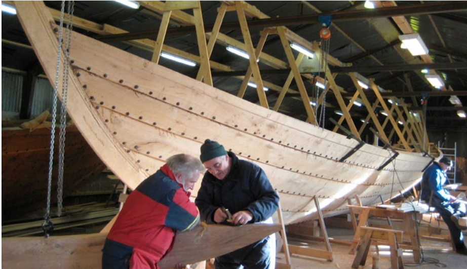
The replica of the 23 metre-long Nydam Boat under construction (all photos courtesy of the Nydam Society).
